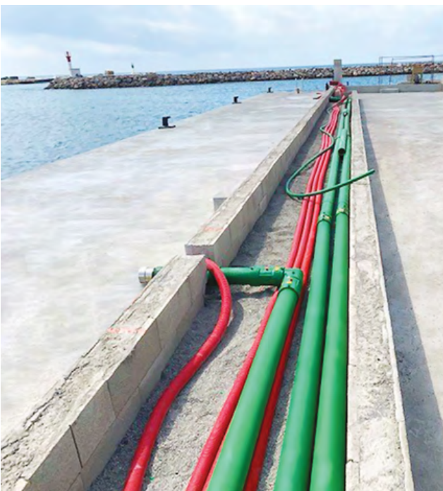
KPS 4" double wall pipe (125/110mm) provides a 933 litre/min flow rate
