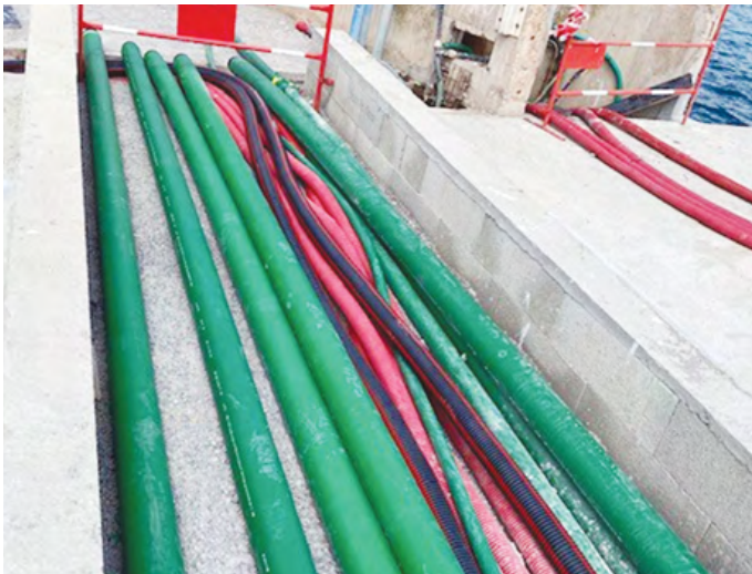
KPS piping includes an EVOH permeation barrier and a conductive layer of carbon black
