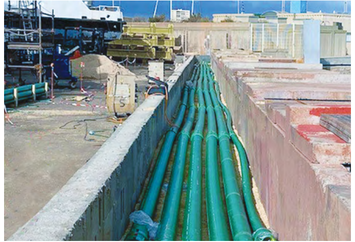
KPS double wall pipework includes an interstitial space between the inner and outer pipes, providing an extra layer of security
