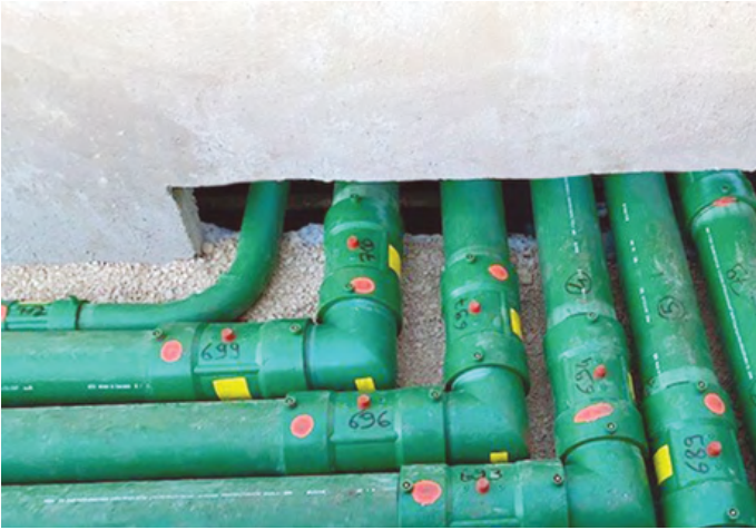
KPS 4" double wall 90° pipe elbows are a compact solution for projects where space is tight
